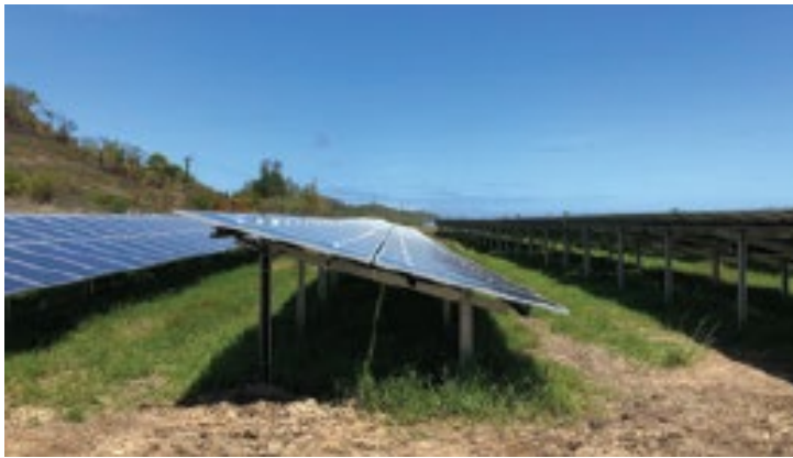
Figure 10 - Dual post pier of racking system (Source: Burgess et. al., 2018)
